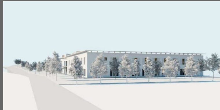
RSA Lavoria -Work in progress-
